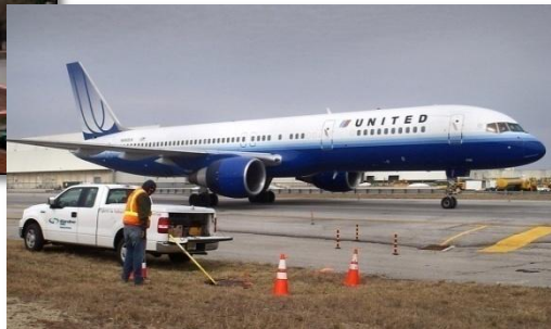
Subsurface Utility Engineering, JFK International Airport, United States
