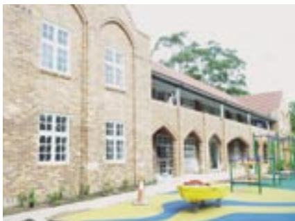
Above: Construction on the Knox Grammar School
