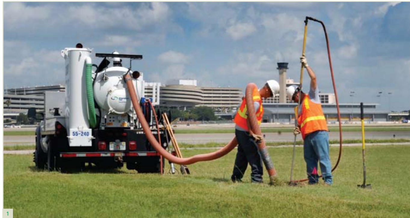
1 Subsurface Utility Engineering Services, Tampa International Airport, Cardno TBE
