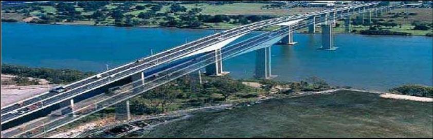
Gateway Bridge Duplication, Qld
