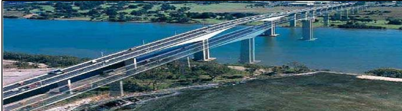
Gateway Bridge Duplication, Old, Aust
