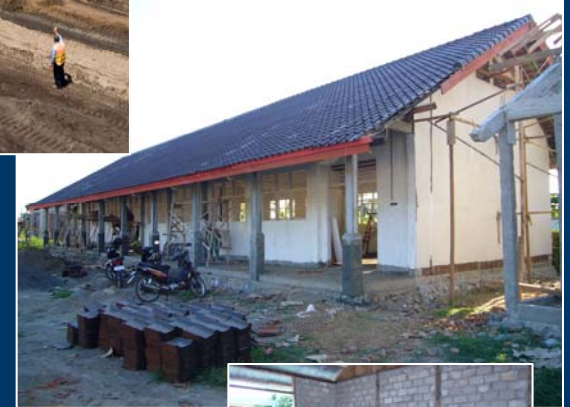
Schools rebuilding program, Indonesia
