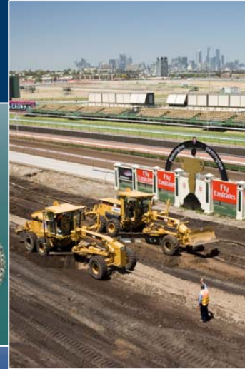
Design & Upgrade of Racecourse - Flemington, VIC
