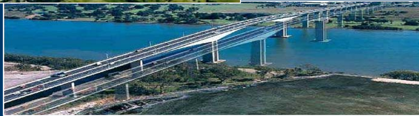
Gateway Bridge Duplication, Qld
