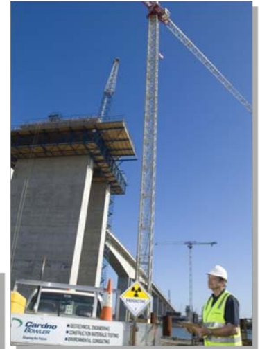
Gateway Bridge Duplication, Queensland
