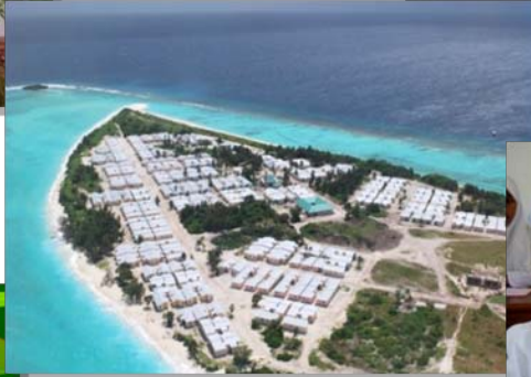
Post-Tsunami Reconstruction Works, Maldives
