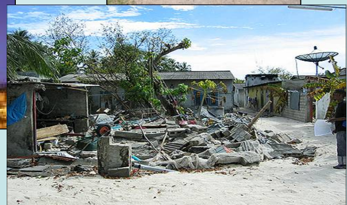
Post Tsunami Reconstruction Works, Maldives
