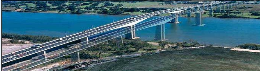
Gateway Bridge Duplication, Old, Aust
